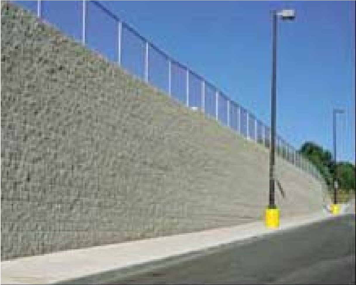
TYPICAL SMALL BLOCK (KEYSTONE) WALL
