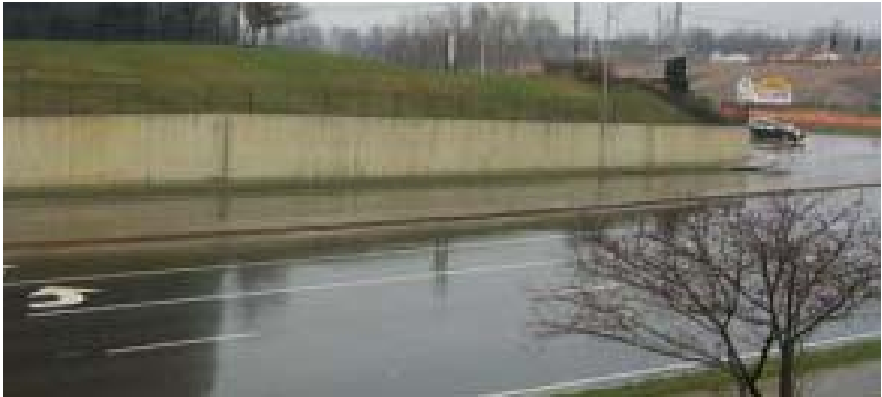
TYPICAL GRAVITY WALL
